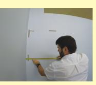
Mark the position of panel '1' using your measuring tape or ruler. Use small pieces of masking tape that will act as guides. Correct positioning of panel 1 is important.
